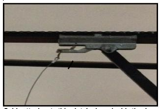
Cable attaches to this clutch gizmo inside the door. It releases the door from the electric opening mechanism. You have to reset the clutch gizmo and put the lock back to restore normal service.
