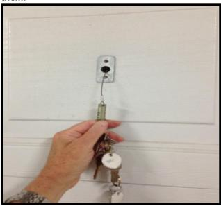
Second: Put key into your well-lubricated and maintained lock tumbler (see article!) and turn one quarter turn, then pull out the lock tumbler, and, finally, pull on the cable to release the door.
