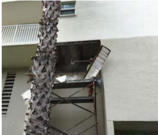
*Above: Work began on fixing Building 7's mysterious dissolving soffit on May 18. The theory is that condensation from the pipes within collected on the covering, which is basically wall-board, and, over the course of 10 years, dissolved same. The new job will be better vented.*
