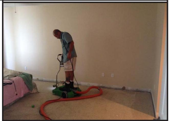
**In flooded condos, soft flooring and baseboards are removed, holes are drilled in the walls to remove water trapped inside them. Photos courtesy Harry Holmgren.**
