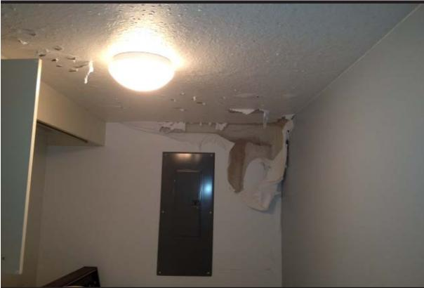
**Ceiling of apartment 3-803. The burst hose sprayed the walls..**
